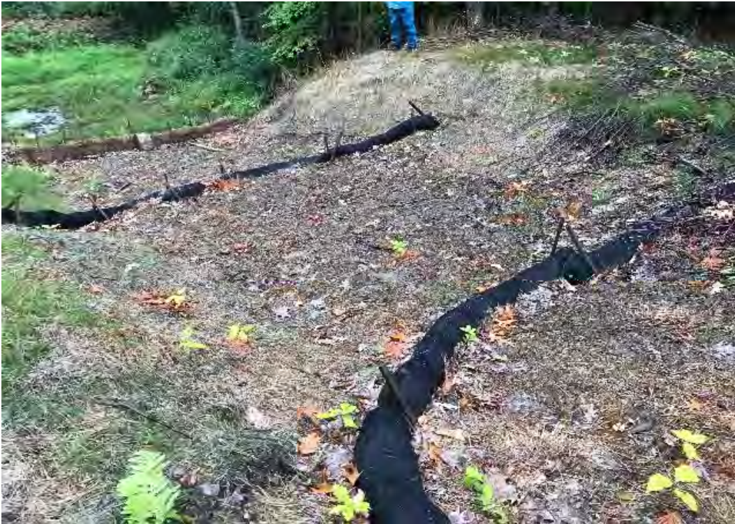
Fig 11: BMPs on the slope between Strs. 29 and 28 are functioning. Viewing north. (08-29-20).
