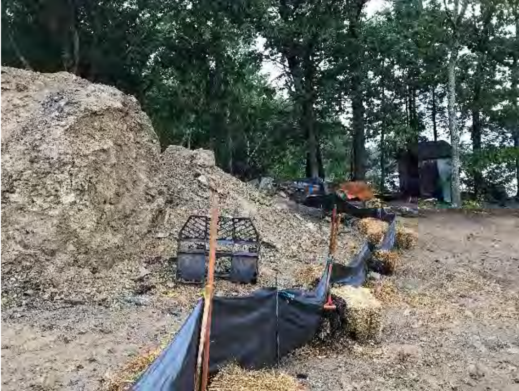
Fig 7: The BMPs stabilizing the soil stockpile at the Eversource property/west side of the bay are functioning. Viewing north. (08-29-20).
