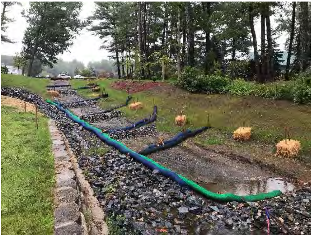
Fig 2: Slope above the manhole at Gundalow Landing/east side of the bay. Viewing east. (08-29-20).
